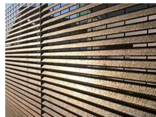
2 METAL LOUVER SCREEN WALL
